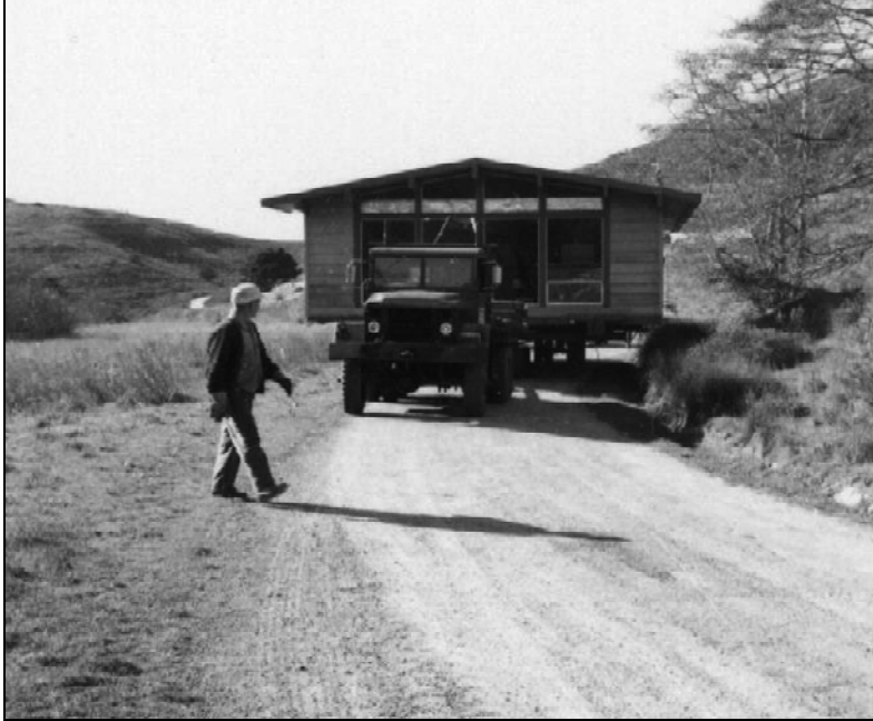
Maintenance crew moves a house from Limantour Spit to its new role as Bear Valley Visitor Center, 1971.
